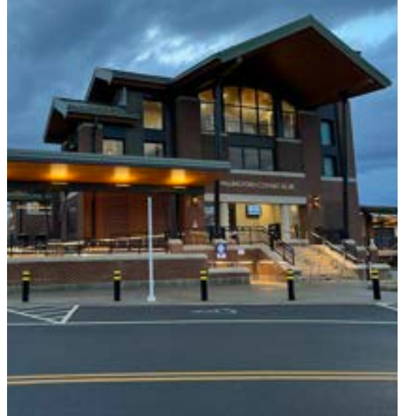
Wallingford Train Station
